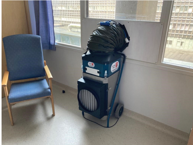
Fig 1. Temporary high-efficiency particulate absorbing filter in place to create a negative pressure environment.
