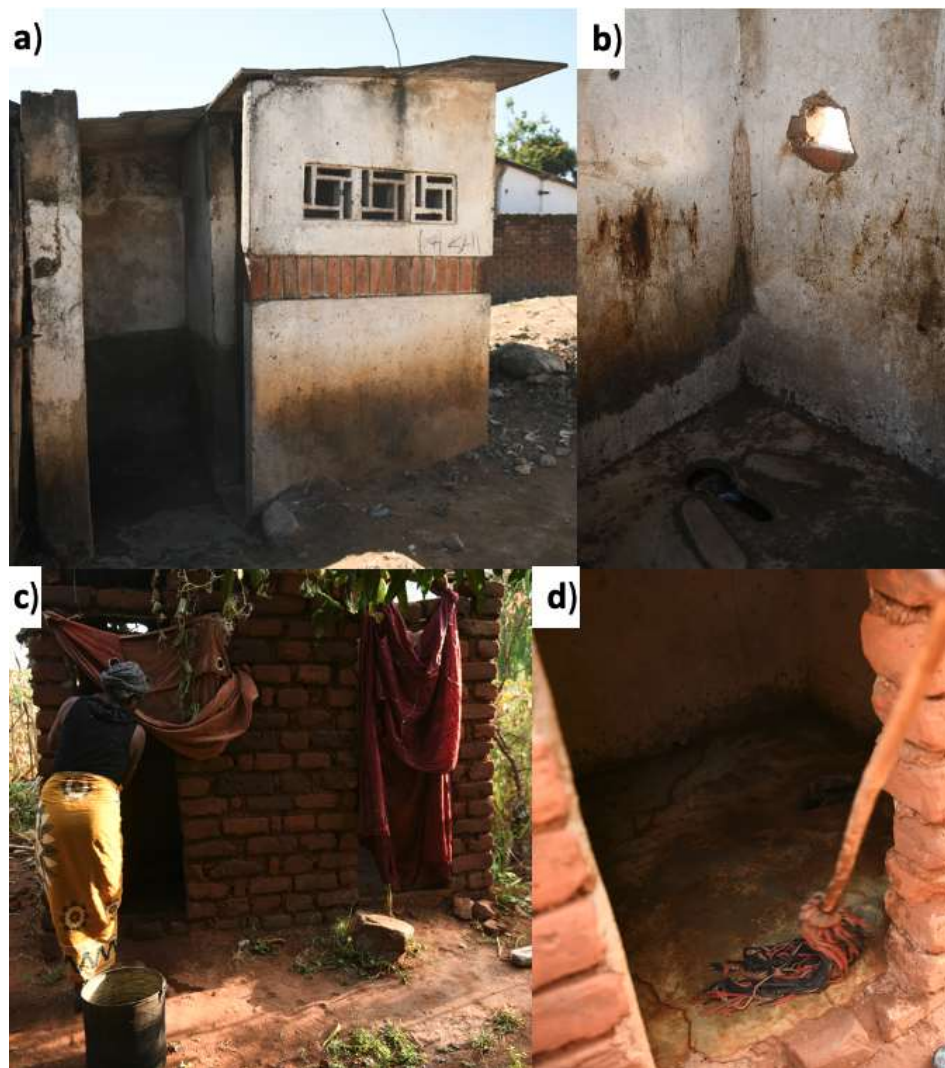
Figure 4.4. Pictures of typical pit latrines used by households. a) external structure of pit latrine in the [urban], b) internal structure of pit latrine [urban], without drophole cover in place, c) external structure of pit latrine [peri-urban] and d) internal structure of pit latrine [peri-urban], without drophole cover in place. Photo credit = Thoko Chikondi, collected as part of Wellcome Trust funded DRUM photojournalism project, June 2021.
