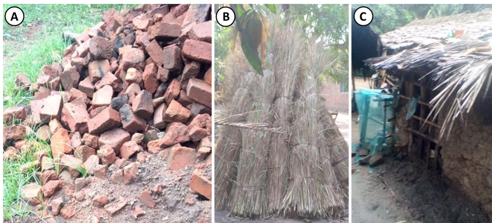
Fig. 6 Examples of readily available traditional construction materials in and around environment of the recruited houses. A Remaining bricks and brick rubble left over after construction of a house. B Bundles of grass thatching collected nearby, which are commonly used for roofing. C Palm leaves used to roof a small mud and wattle house
