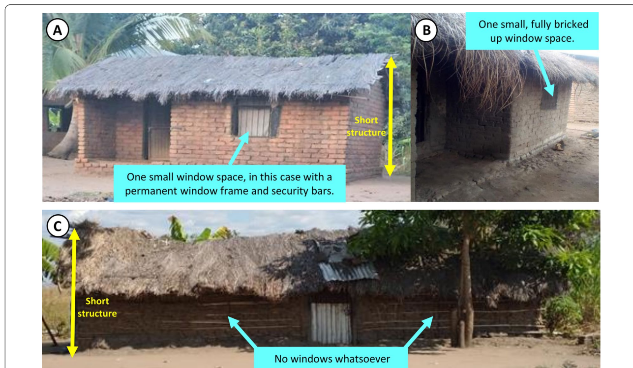
Fig. 5 Representative examples of the cluster one houses with poorly planned ventilation based on traditional designs, which were often built with traditional materials like mud and wattles or unbaked bricks for the walls and grass thatch or palm leaves supported by bamboo poles for the roofs
