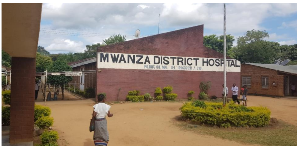
Figure 14: Front view of Mwanza District Hospital
