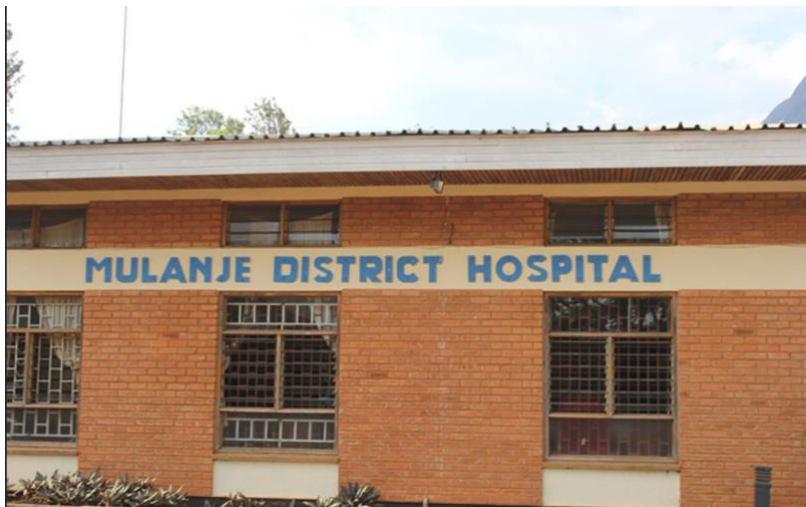
Figure 15: Side view of Mulanje District Hospital
