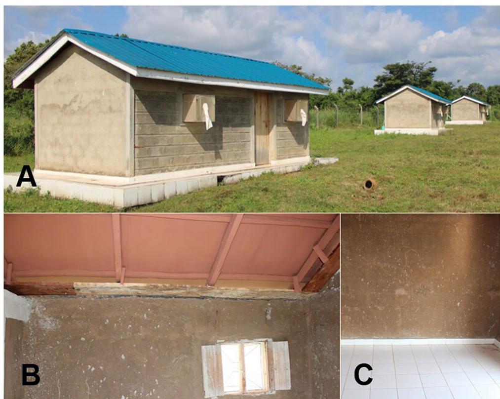
Fig. 1 Experimental hut design: A front view of the hut fitted with window exit traps, B showing the tiled floor and the hut interior walls and C showing the wood baffles
