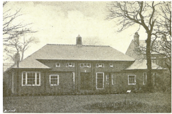
THE NEW DISPENSARY, MILL LANE.
